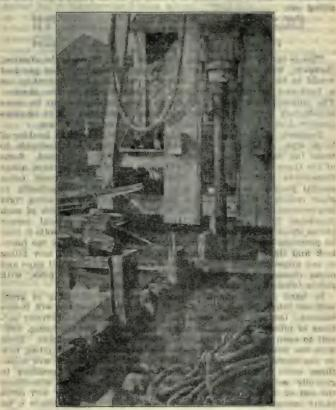
Fig. 5.-View Showing Arrangement for Driving Steel Sheet Piles. (A) Bottom of Steam Hammer; (B) Wooden Block; (C) Cast Iron Follower; (D) Steel Pile.
